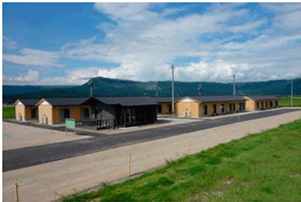
Example of constructed temporary housing (wooden)
