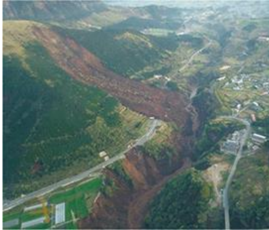
Slope failure in the area where the Aso-ohashi Bridge stood
