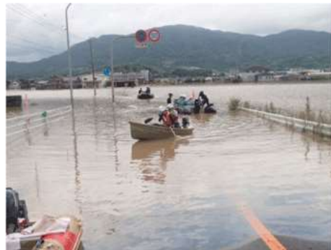
Inundation in Saga Prefecture (Tekeo City) (Source: Cabinet Office)
