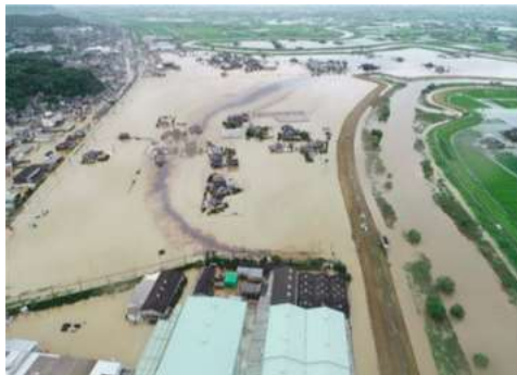
Inundation in Saga Prefecture (Oomachi Cho) (spillage of quenching oils) (Source: Ministry of Land, Infrastructure, Transport and Tourism)
