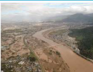
Damage at Nagano City, Nagano Prefecture
