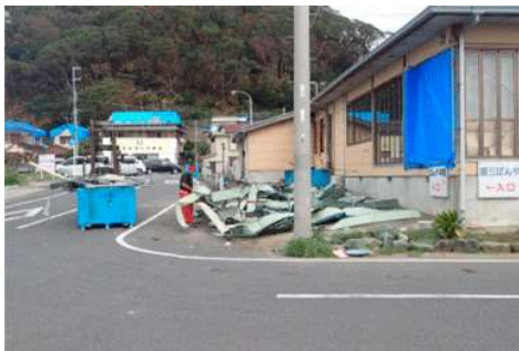
Damage to houses in Chiba Prefecture (Kyonan Town) (Source: Cabinet Office)
