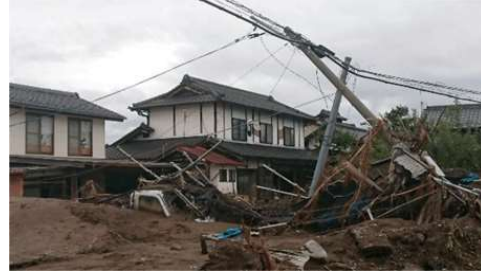
Sediment disaster in Nagano Prefecture (Nagano City) (Source: Cabinet Office)
