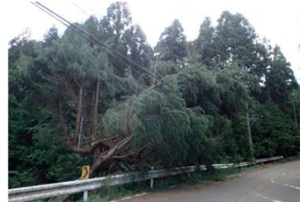
Damage caused by fallen trees in Chiba Prefecture (Katori City) (Source: Cabinet Office)
