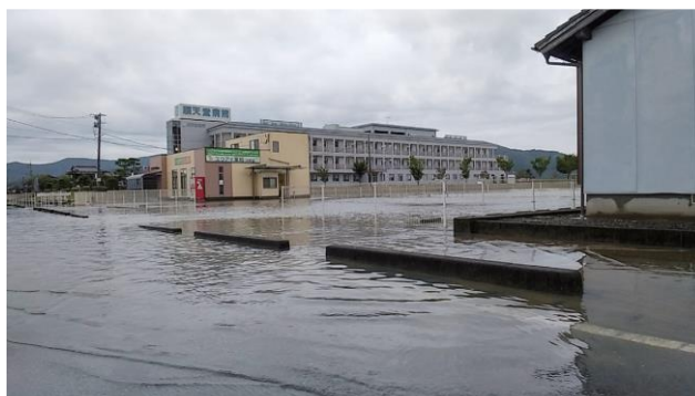
Flooding damage at Rokkaku River in Takeo City, Saga Prefecture (Source: Cabinet Office data)
